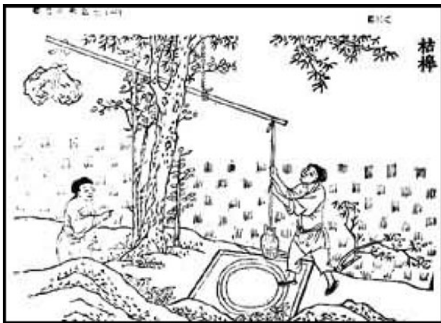
Fig. 4 Shadoof used in ancient China, adapted from Zhou 2008
